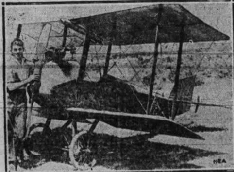
**"BABY" PLANE RACE ENTRY**—A baby aeroplane, which weighs but 228 pounds, has been entered in the race for light planes to be held during the International Air Races at Dayton, O. It has a wing spread of twelve feet and is propelled by a sixty-one cubic inch displacement motorcycle engine. Bert Mix, an aeroplane mechanic of Dayton, built the machine, which can make about seventy-five miles an hour.
